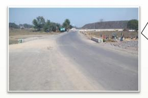
Construction of Road from NH to Old Munda Basti with project cost Rs.41.00 lakh has been completed. The road connecting to Munda Basti is the end of Municipal area morum metal road. Now it has been constructed with bitumen road providing guard wall on both side of the road, which will serve as all whether road.
